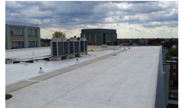
Source: Philadelphia Water Department, "Blue Roofs"
