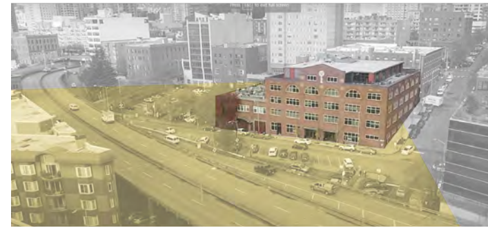
Before demolition, view of Western Ave from west:
