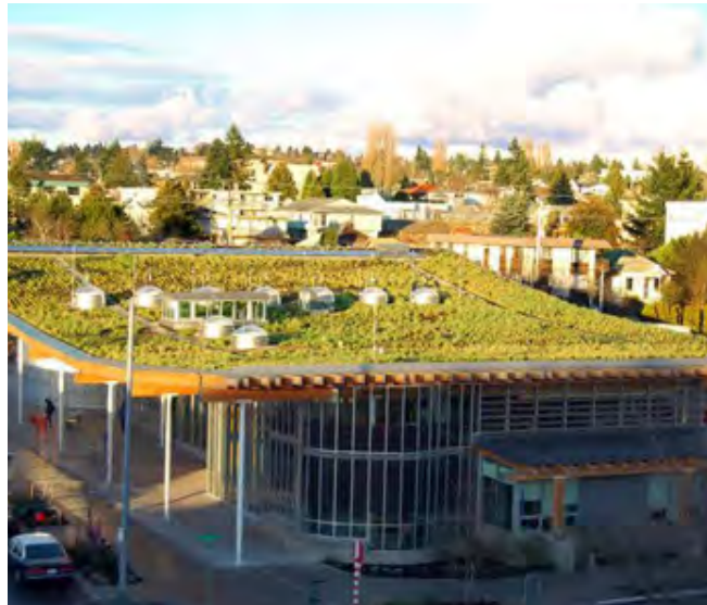
Source: My Ballard, "Seattle's rooftops are going green"
