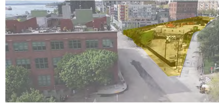
After demolition, view of Western Ave from south:
