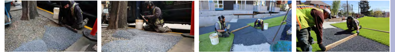
Process of implementing porous treepit material Credit: RootCauseSeattle.com
