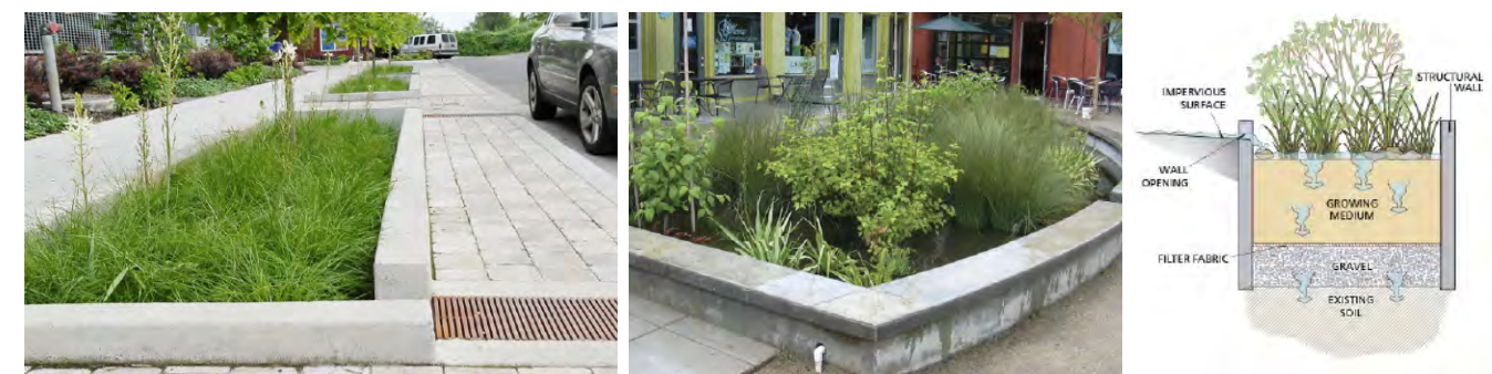
Left: Beaumont Village Lofts (Portland, OR) / Middle: Mississippi Commons (Portland, OR) / Right: diagram of infiltration planter Sources: City of Portland Environmental Services & Clean Water Services
