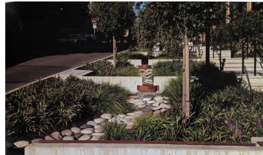
STORM WATER MANAGEMENT - BIORETENTION CELLS AND RAINWATER CATCHMENT GARDENS USED TO CAPTURE AND CLEANSE STORM WATER
