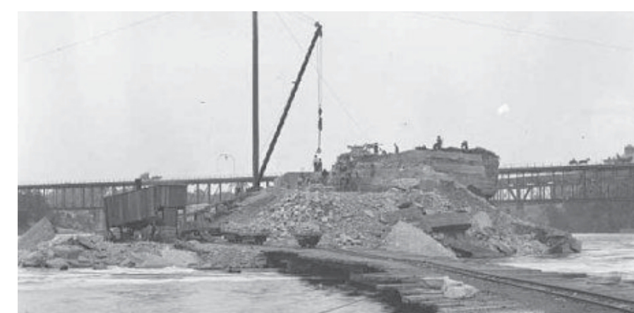
Spirit Island, 1960, Source Unknown; Spirit Island was dismantled by the Army Corp of Engineers to dredge boat passage to the lock and dam.
