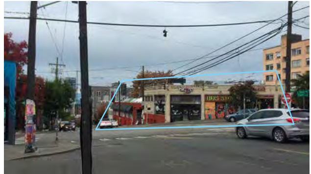
THE BUILDING FACADE IS DETERIORATING
