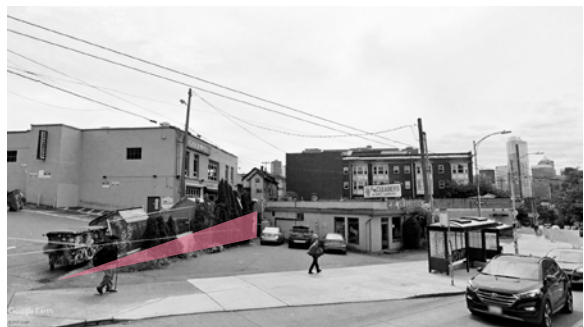
Drop in elevation from alley to adjacent lot.
