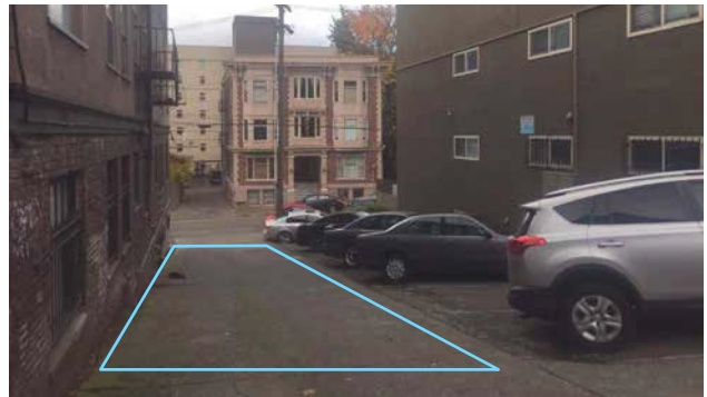
THE PAVING IS NOT PERMEABLE
