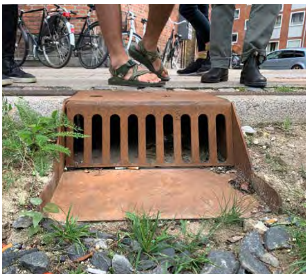
Inside the drain from sidewalk to swale PHOTO BY KRISTA DOERSCH
