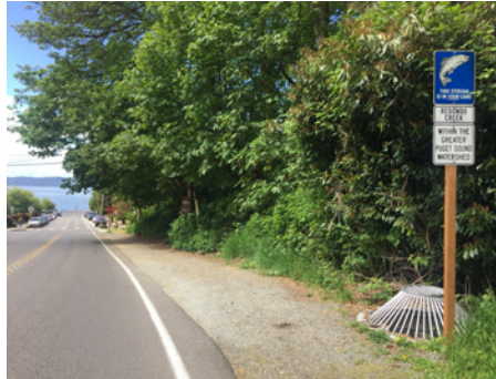
Existing Buried Redondo Creek Drain
