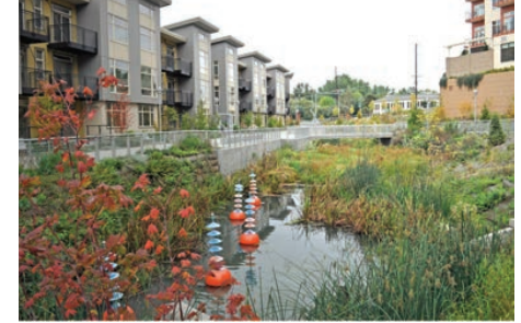
Thornton Creek Water Quality Channel, Seattle
