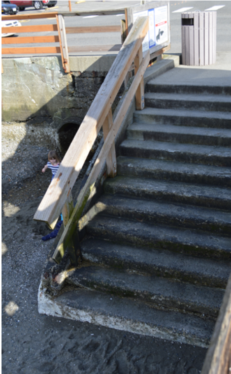
Existing Staircase Used To Access Reef
