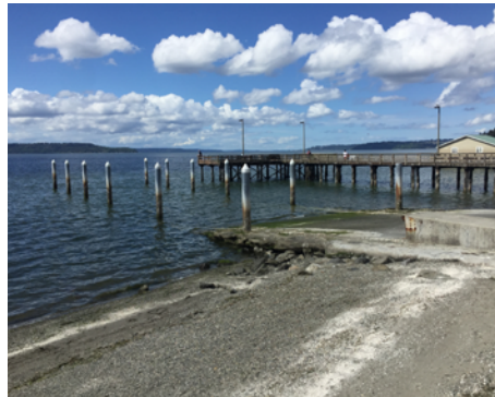
Existing Boat Launch and Fishing Pier
