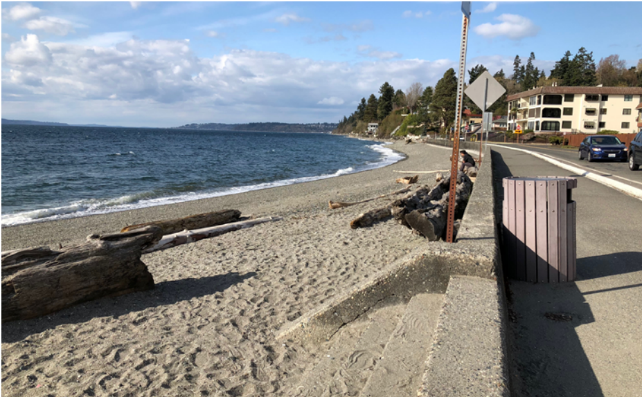
Existing Access Point Over Sea Wall
