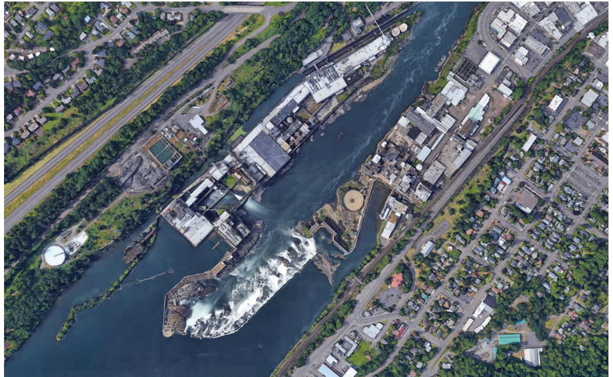
Figure 3, top: Existing conditions, aerial
