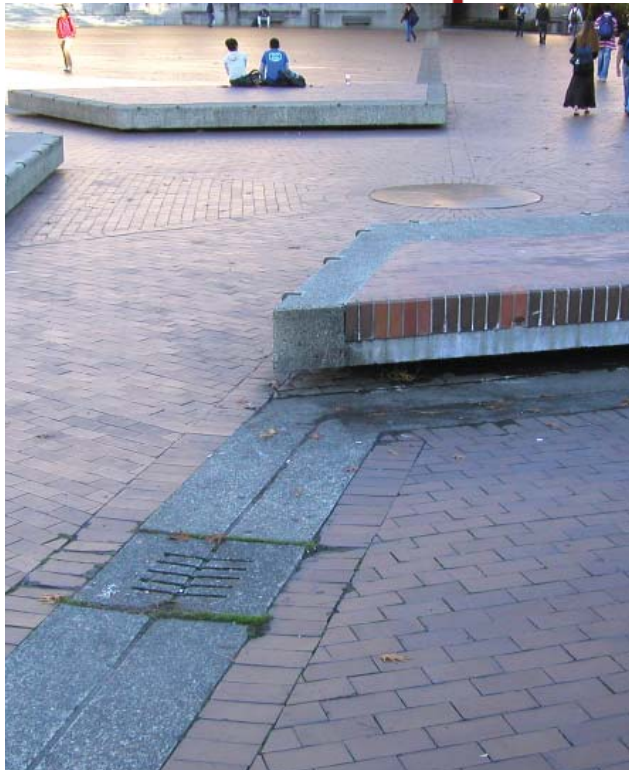
catch basin in plaza
