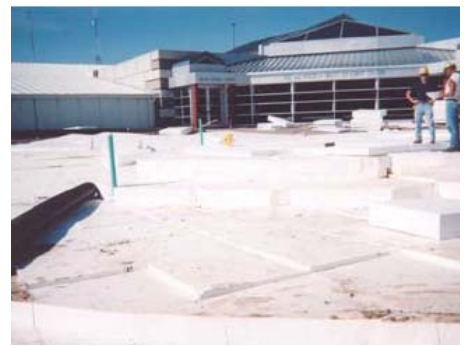
geofoam was used to elevate this plaza grade in a limited live load situation
