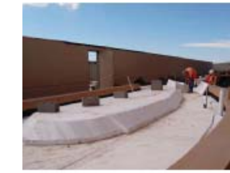
geofoam used as lightweight fill in a rooftop application
