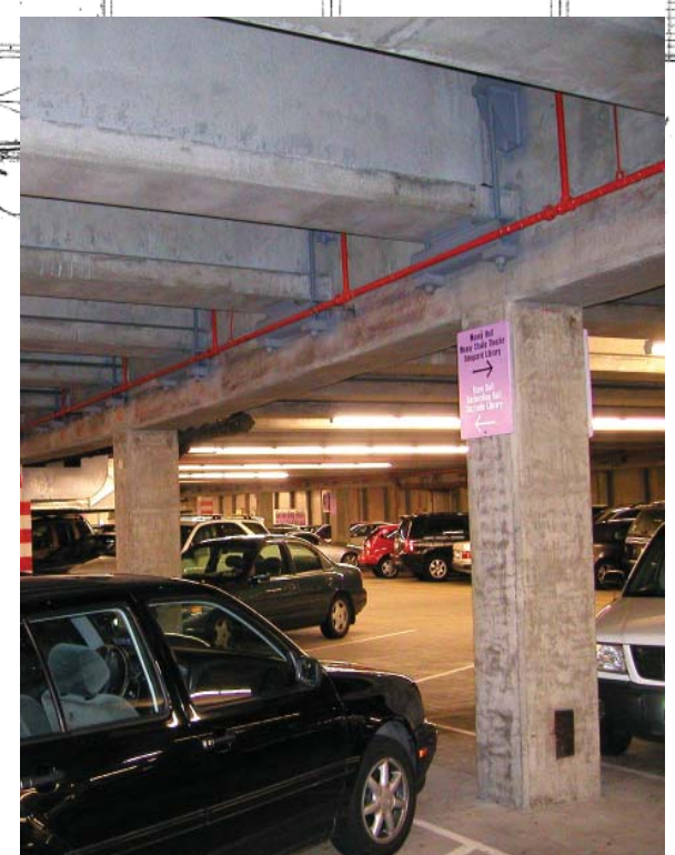
concrete columns and beams
