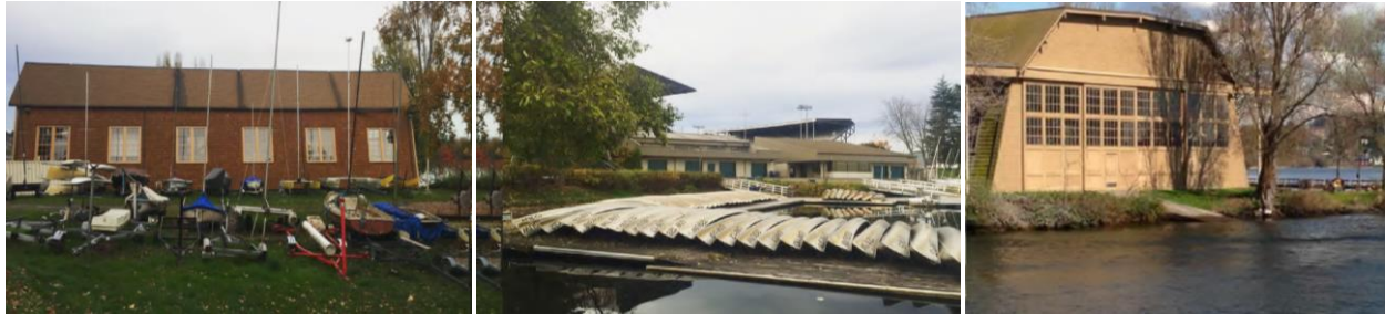
UW Canoe House and Water Activities Center, Montlake Cut
